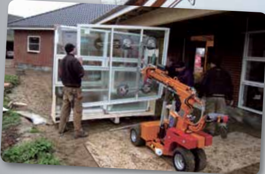
The wide tyres make the lifting device suitable for difficult off-road jobs.
